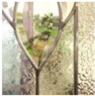
Zinc Caming Standard Low-E with Argon
